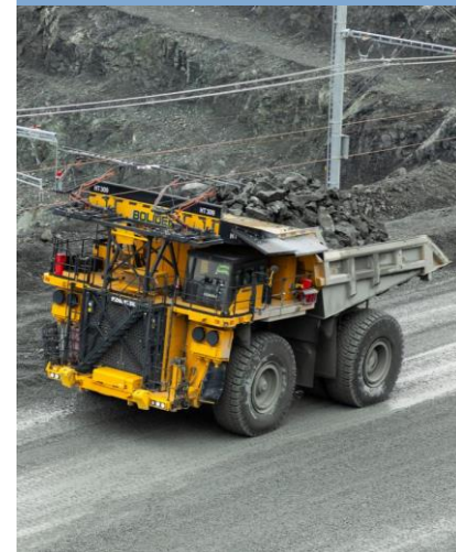
Electric trolley line in Kevitsa
