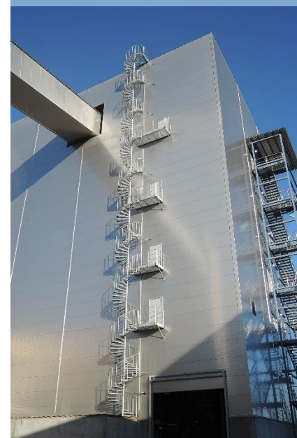
Harjavalta, sulphuric acid plant.
